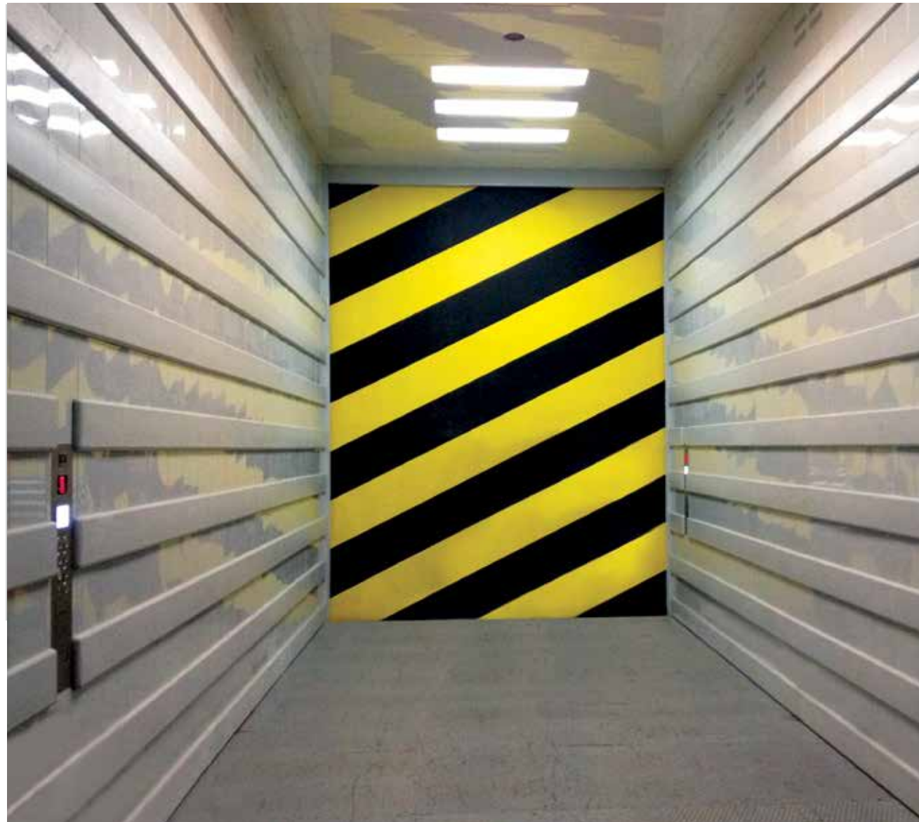
Custom-made Hydraulic Freight Lift 3,6 m wide x 8m depth x 4,7 m height
